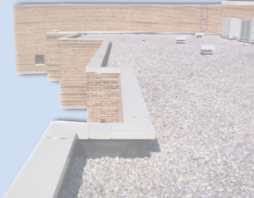
FiberTite Coping Tapered, Flat or Existing Versions 24ga., .040", .050", .063" coping cover
