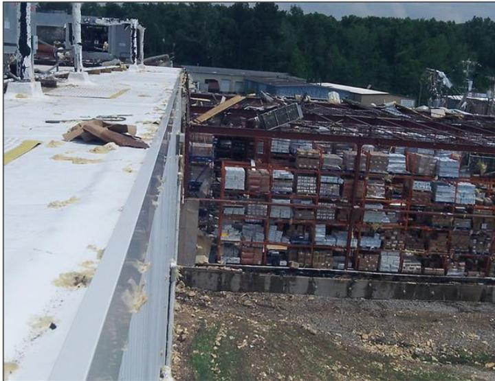
The building shown on the left installed Edge Systems One Fascia by Metal-Era. When an F3 tornado hit this US Foods Warehouse in Pearl, MS the building with Edge Systems One was still intact while the other building suffered complete failure, causing significant damage.
