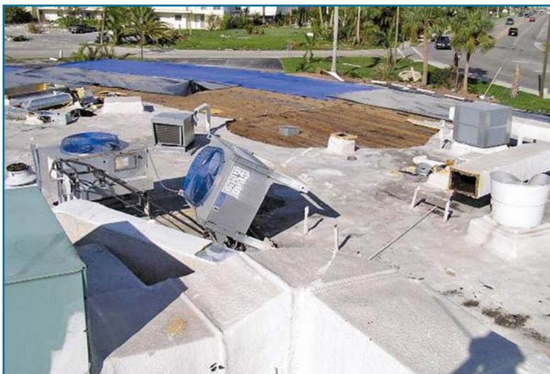
*Figure 1 – Hurricane Charley, 2004: Edge flashing damage initiates roof blow-off. Photo courtesy of RICOWI.*
